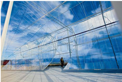
“enclosed trough” for enhanced oil recovery . Photograph: GlassPoint Solar
