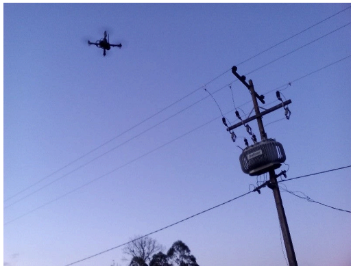
Fig. 9. Visual inspection with the prototype seen from the ground
