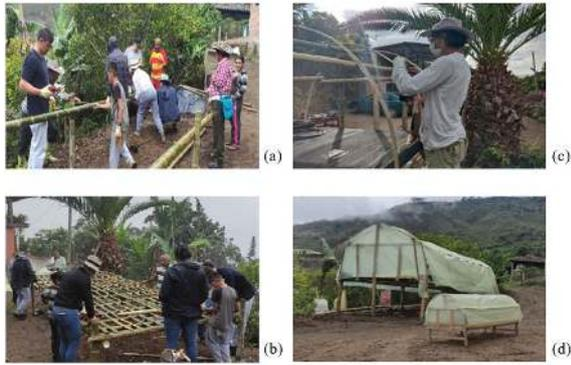
Fig. 8: (a) Foundations and footings; (b) Lateral supports; (c) Arch construction; (d) Installation of plastic lining.
